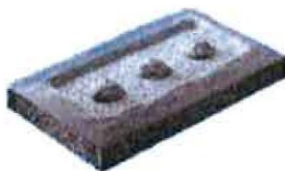
Figure 1. Applying adhesive to the thermal insulation panel
